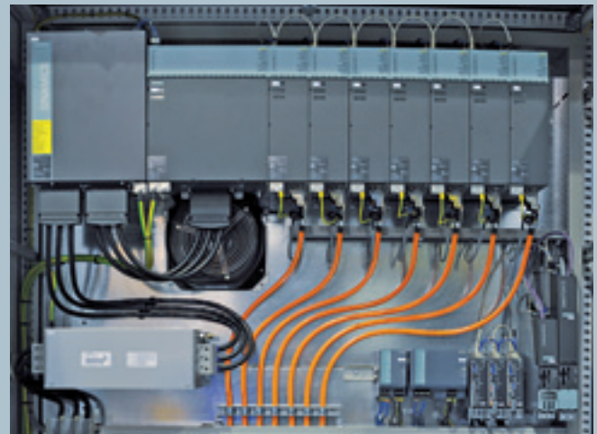
Control enclosure of the Maxis SI with SINAMICS S120 components and SIMOTION D motion controller (lower right)
